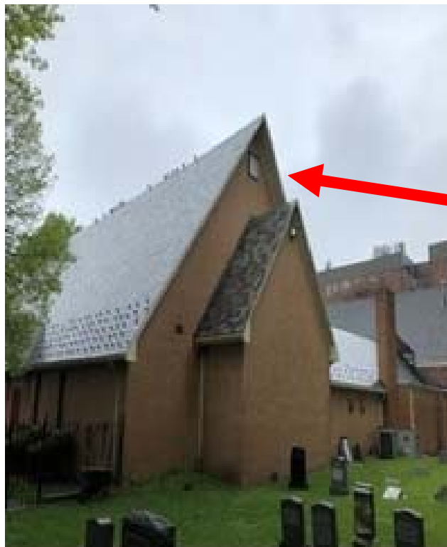
Attic or Cockloft Vent (Photo 1B)
