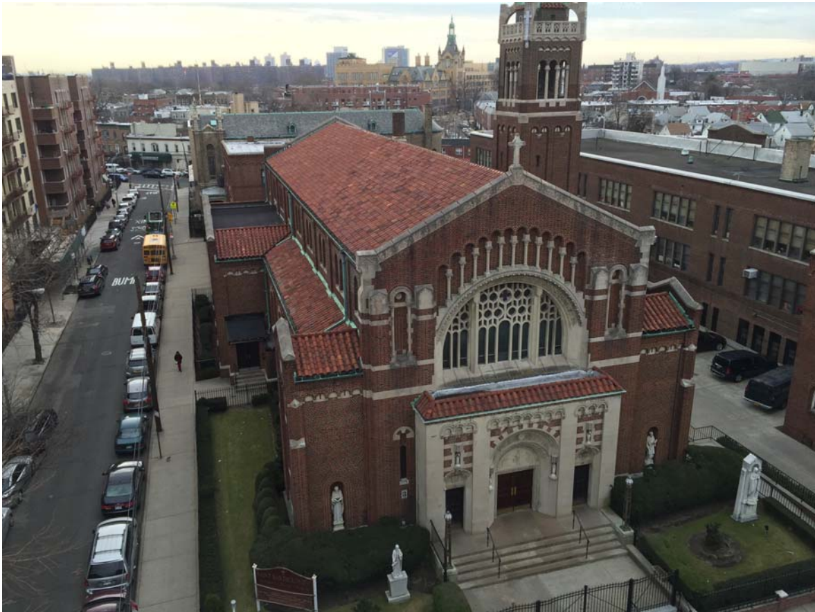
Roof Coverings (Slate/Terracotta tiles) add significant Dead Load. In addition, TL stream may dislodge tiles and cause injury (Photo 20)
