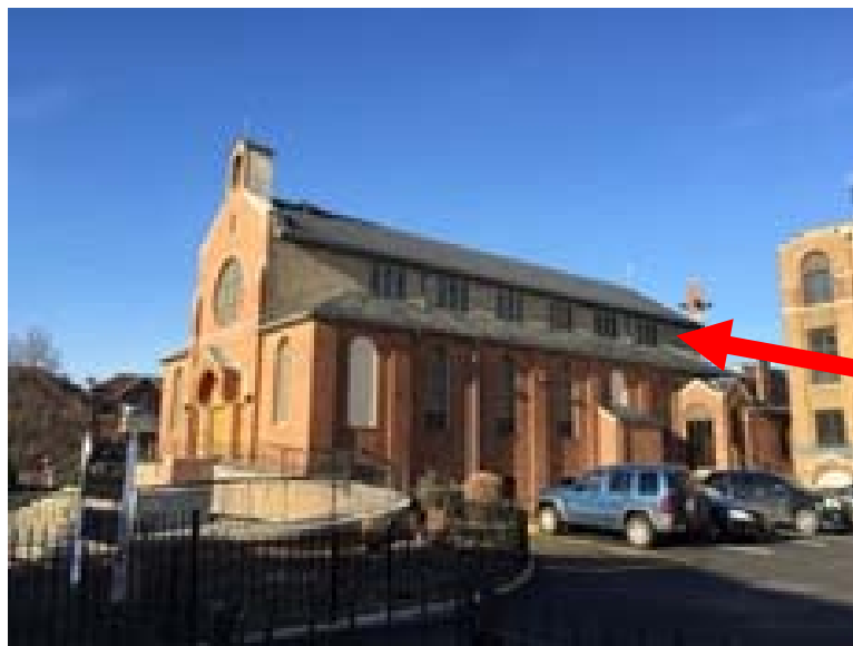
Clearstory Windows (Photo 5)
