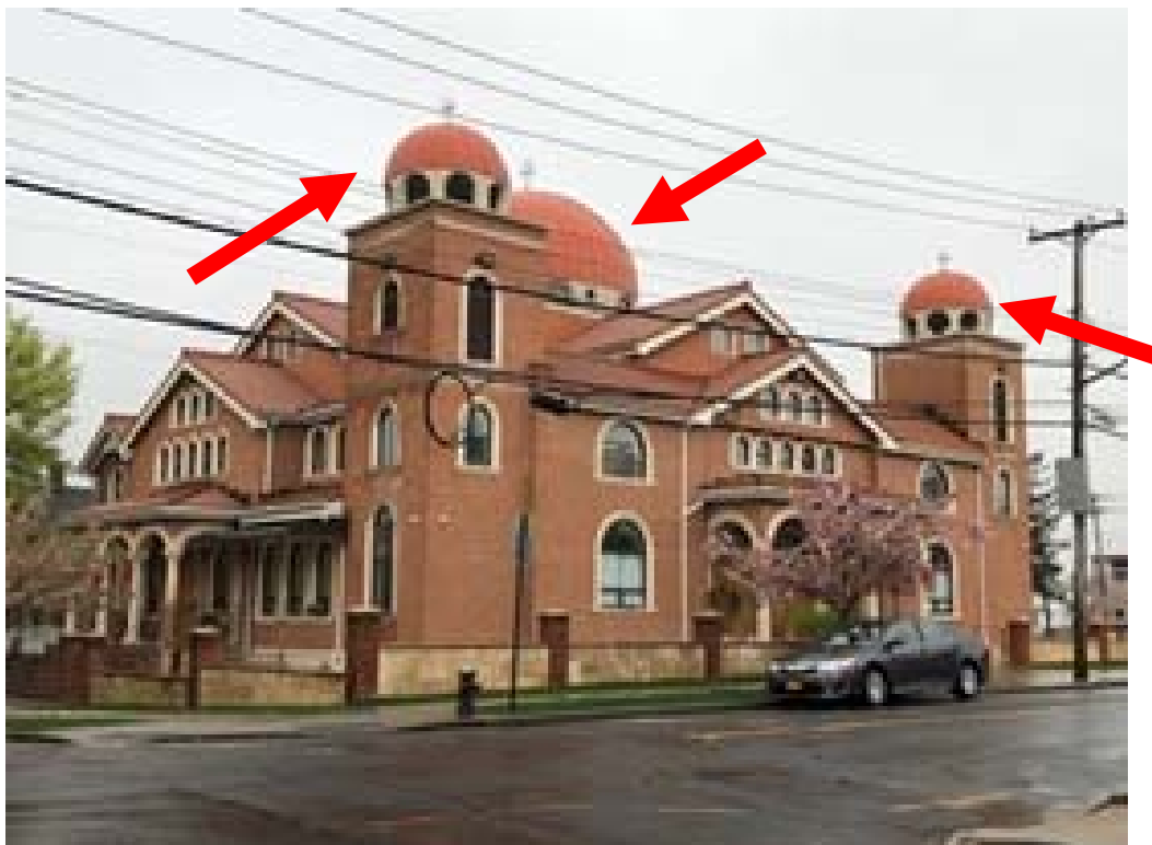
Masonry Domes (Photo 9)
