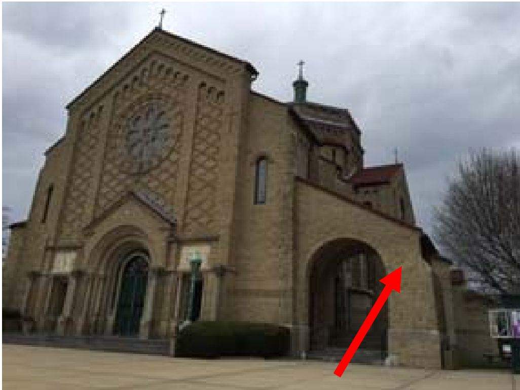
Flying Buttress (Photo 8)
