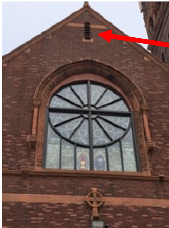
Attic or Cockloft Vent (Photo 1A)
