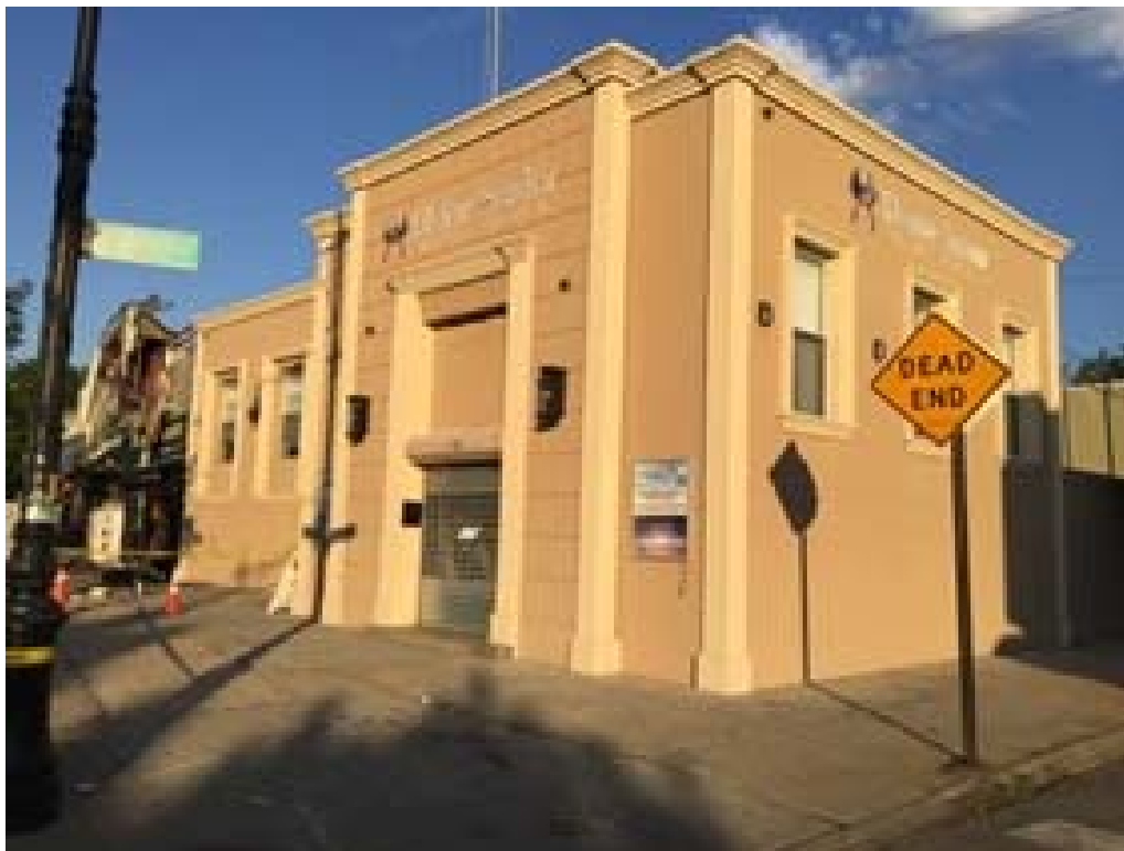
Hazards such as Exterior Insulation Finishing Systems (EIFS) (Photo 17)
