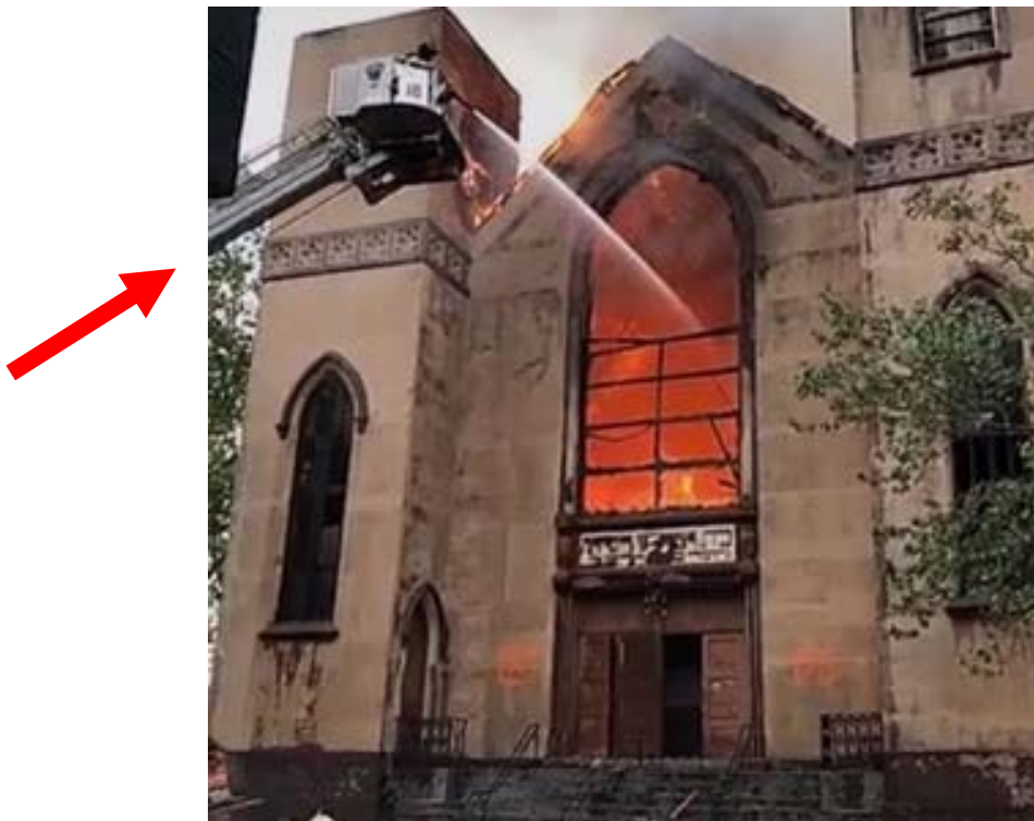
Corner Safe Areas (Photo 7)
