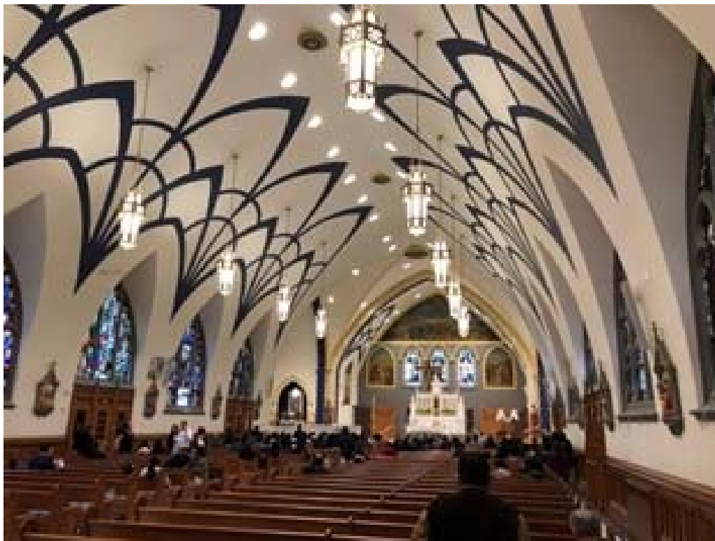
High Vaulted Ceiling (Photo 19)
